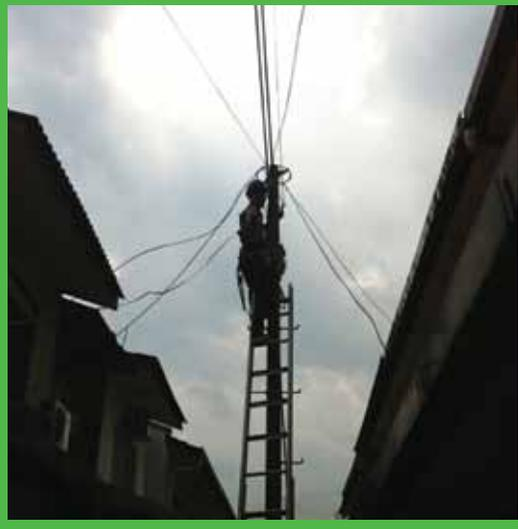
FDP on pole. Installer fixing cable from pole
