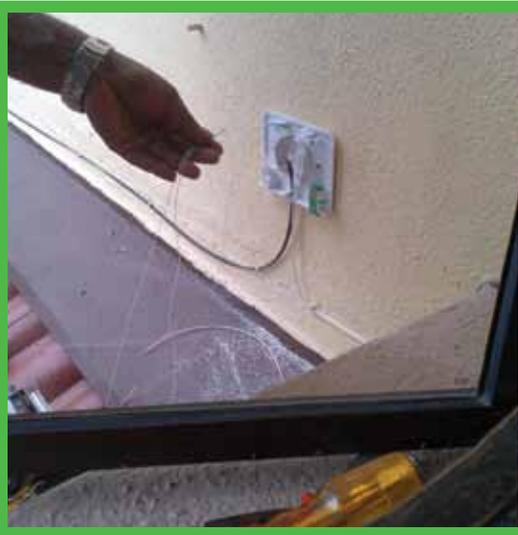
Fibre coiling at FTB
