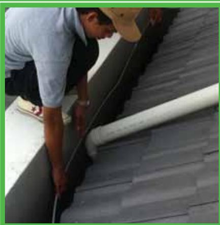
Concealed cable routing with microduct at the edge of roof
