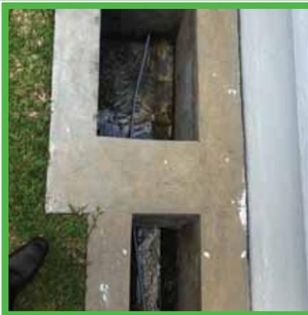
Concealed cable routing through drain (with microduct)
